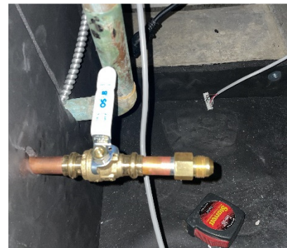
Figure 5 New runout with isolation valve
