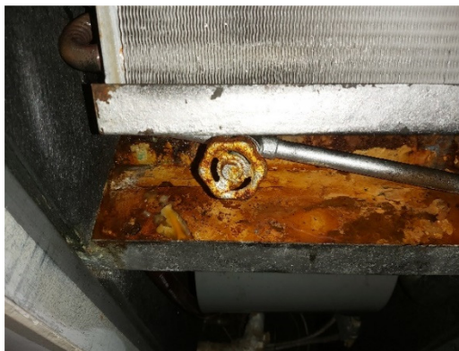
Figure 1 Rusty drip tray and bacterial growth
