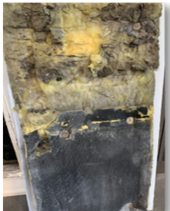
Insulation Deterioration
